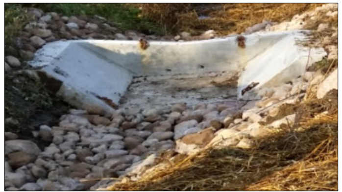
Completed installation of the first pilot sediment trap on Town Hall Road (November 2015).
