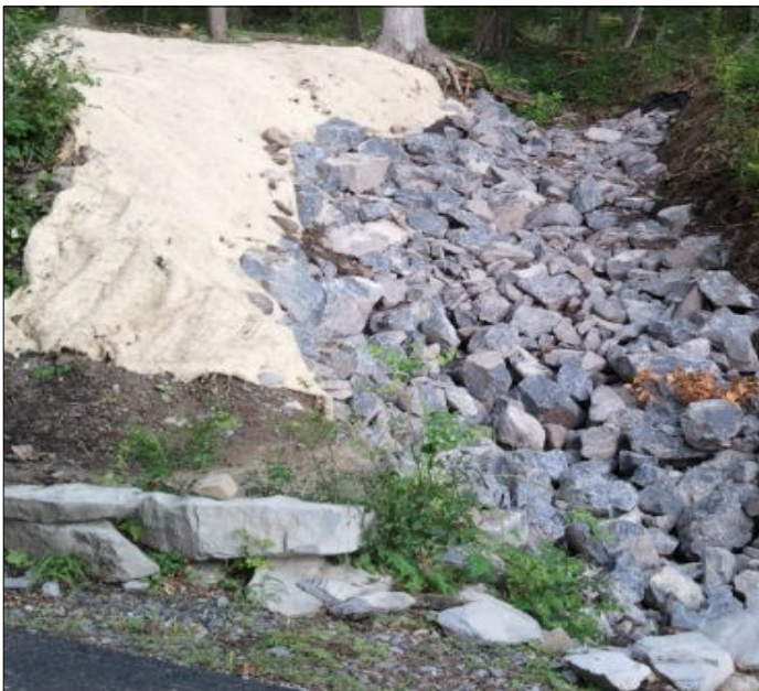
This site on East Lake Road in Owasco demonstrates the use of a variety of erosion and sediment control methods on a severely eroding site. The methods shown in the photo include: a burlap-like rolled erosion product (left), and angular stone protection or "riprap" (right).
