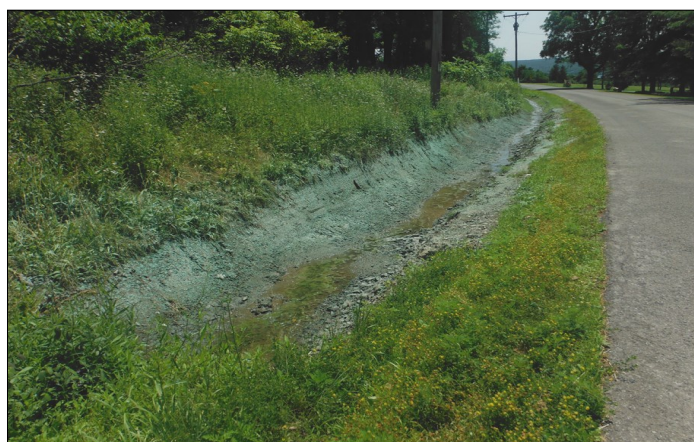
Hydroseeding is an effective and inexpensive practice for stabilizing roadside ditches to minimize erosion and prevent nutrient loading in waterways.
