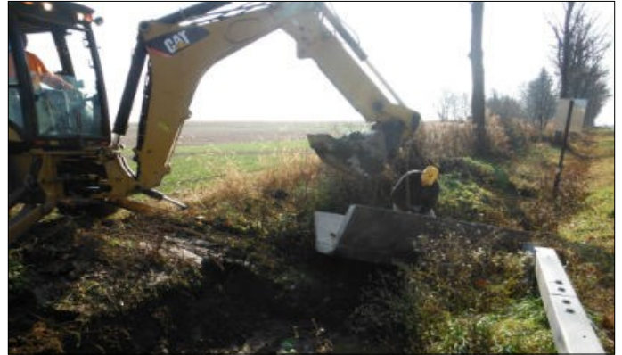
Owasco Highway Department personnel help install the first pilot sediment trap on Town Hall Road.
