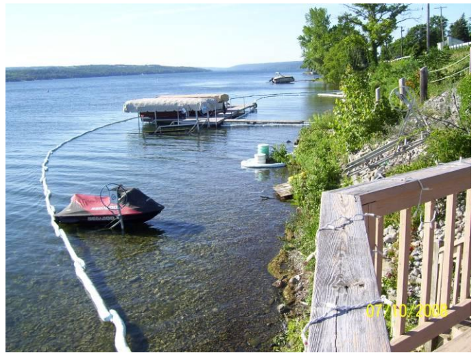
Booms in water to trap hydraulic oil (looking to the south)
